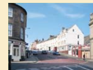
Planning permission for a restaurant and affordable flats was given on this corner site, but it has been sold on and there are now plans for a tall apartment building with ground-floor commercial premises.
